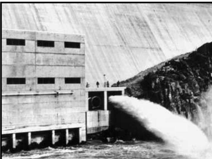
One of two Ring-Jet Valves used for irrigation bypass at Tulloch Dam, California. Shown here at full discharge under 145 feet of head.
