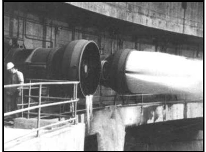
Battery of Ring-Jet Valves controls flow while dissipating energy and reducing spray – even in cold climates.
