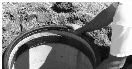
Placing RLA adapter onto riser
