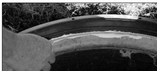
Applying adhesive fillet to inside of riser
